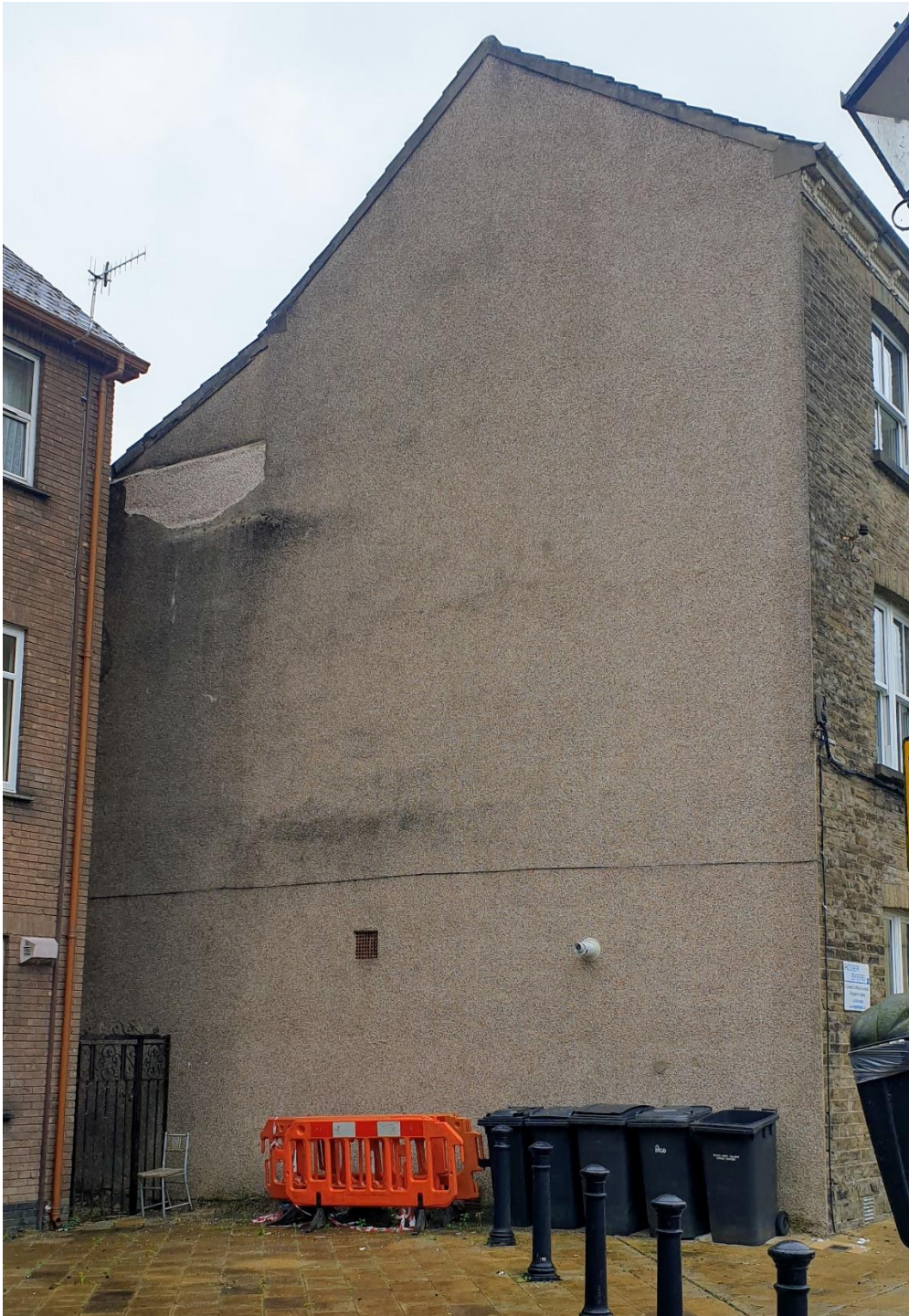
Side elevation (showing repair work)
